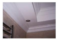
M221 is suitable for most moulded cornices, but adhesion may vary against dense moulds particularly where release agents have been used, heavy moulds, plaster moulds, and PVC faced substrates. Careful evaluation of adhesive properties is essential.
